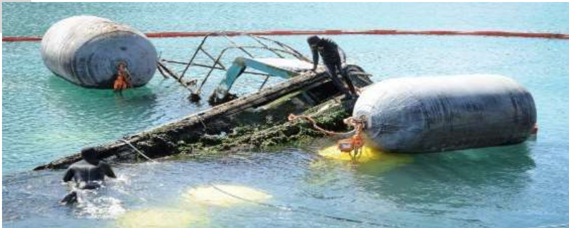
• Process of removing the sunken vessels
