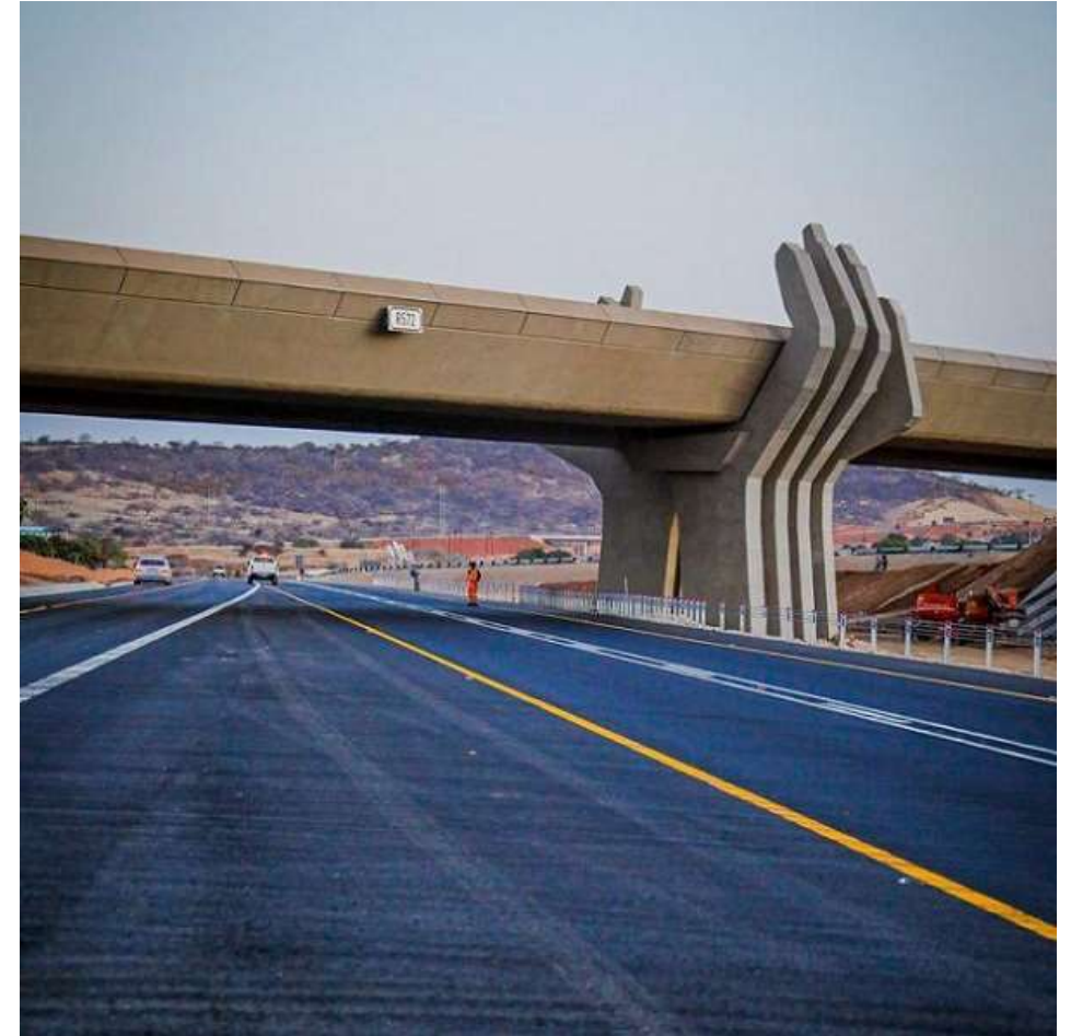
Completed Musina Ring Road
