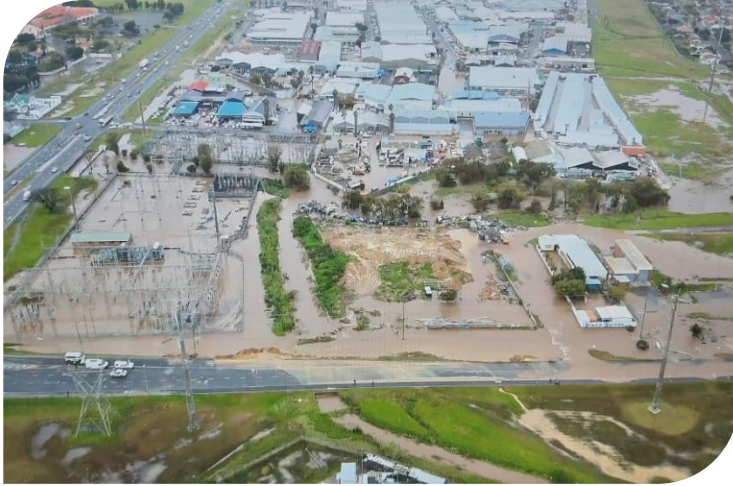
Eskom Substation at Somerset West on Lourens River crossing the N2.
