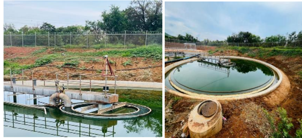
Condition of the clarifier after commissioning
