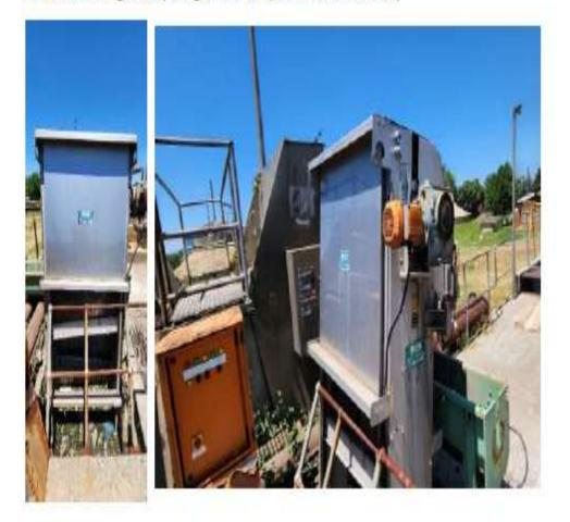
After: Removing and repairing Screen # 4 (Functional Screen)
