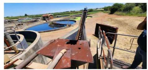
After: Grit Classifiers completed with discharge pipework. (Functional Grit Classifier)
