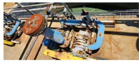
After: New blowers complete with electrical motor. (Functional Blower)
