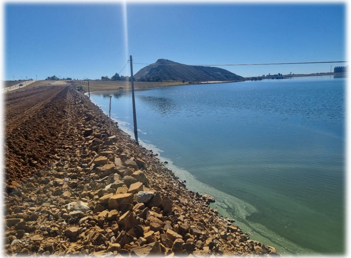
ADDITIONAL ROCKFILL AT VOËLPAN
