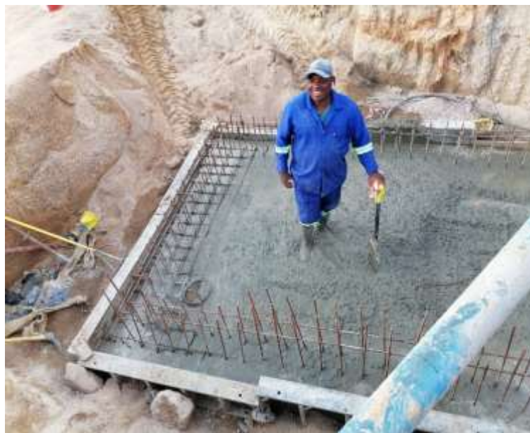
Casting of connection chamber floor slab.
