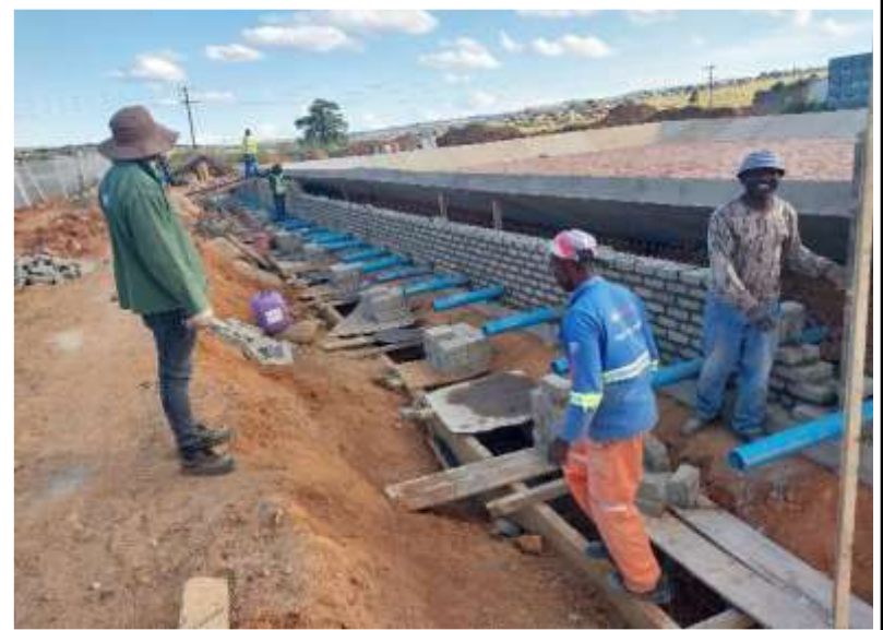
Retaining wall construction
