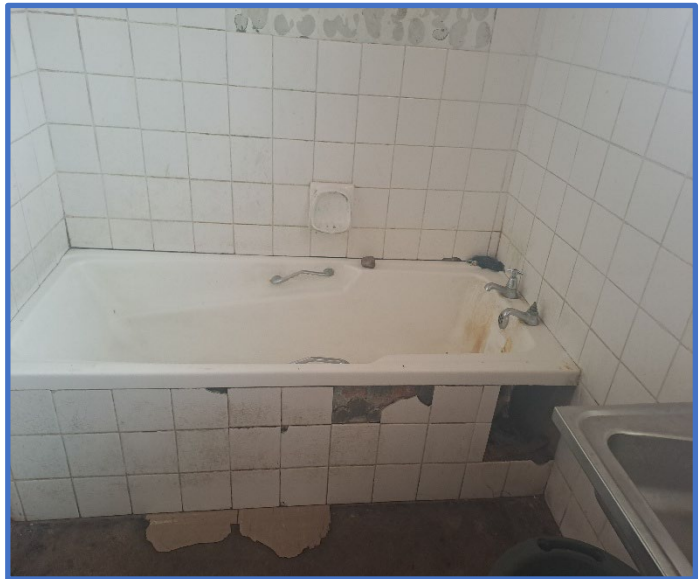
Images 4 and 5: Bathroom Facilities in Domestic Quarters
