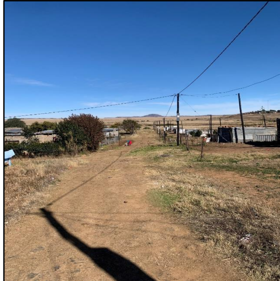
MNG electrification of stands
