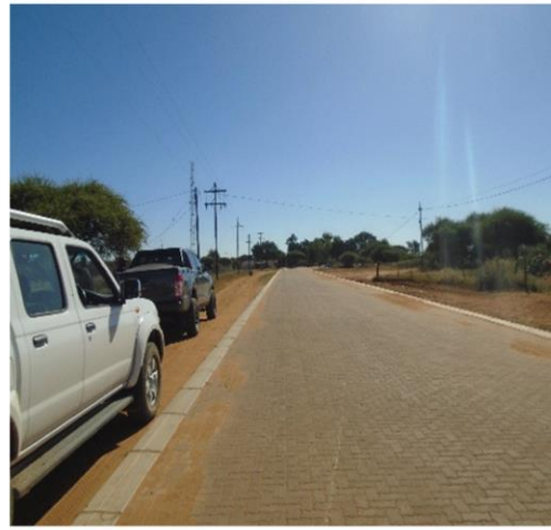
NW: Mahikeng roads construction
