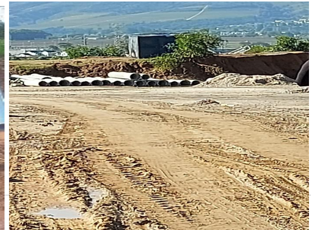
CCT: Macassar bulk infrastructure
